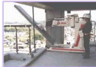
Fig.4. Kajima's interior wall assembly robot
