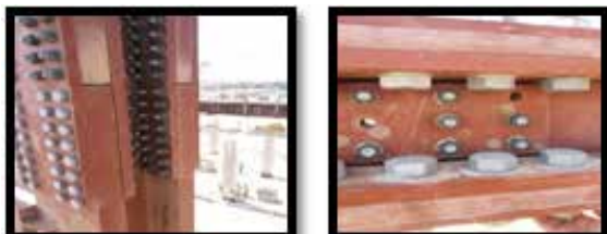
Fig (2) Connection detail for column
