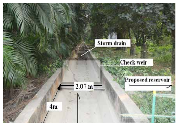
Fig-15: Storm drain carries surplus rainfall runoff
