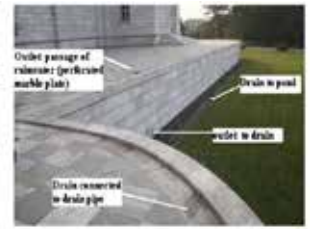
Fig-11: Interconnection of drain to Ponds
