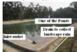
Fig-12: Interconnected pond with inlet/outlet Drain Fig-13: Inlet connection to convey Land scape Drain rain into the pond
