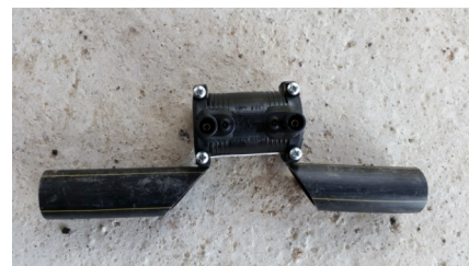
Figure 11. Incorrect Electrofusion Welds For Dn32
