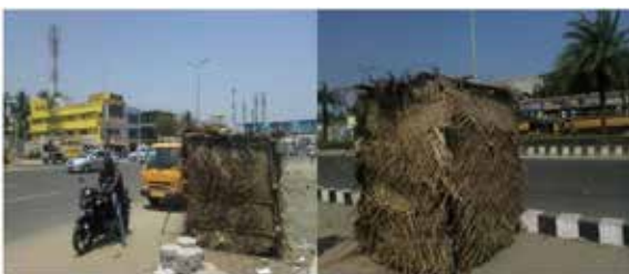
Fig. 2 Noise barrier as a shed at both locations
