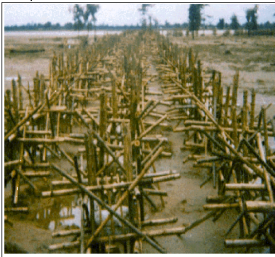
Fig. No. VIII Photograph Showing Effectiveness of permeable spur
