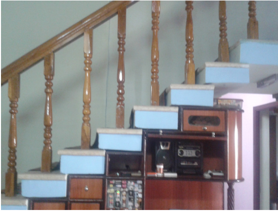
Fig.5: Isolated Steps fixed with wall
