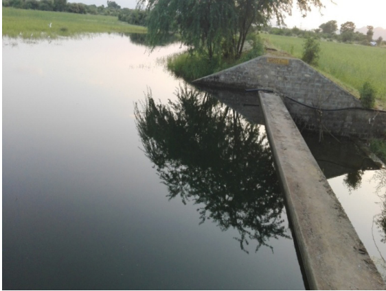
Photograph 2. Masonry dam constructed at village Baitarana near village Ramsin.
