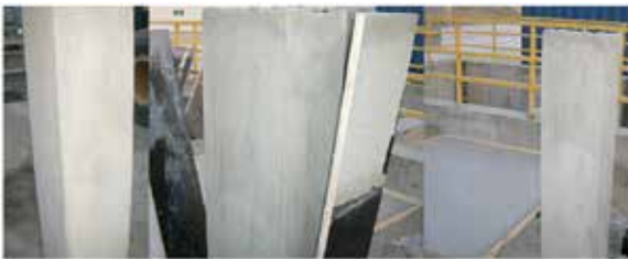
Fig.. 9 SCC Prefabricated elements
