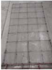
Fig 2. Mesh and reinforcement details of panel
