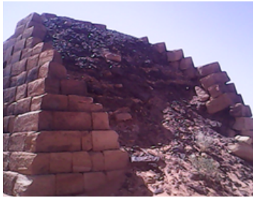
Figure 6: The Structural Function of the Inner Rubble. (Photo taken by Author (2015))
