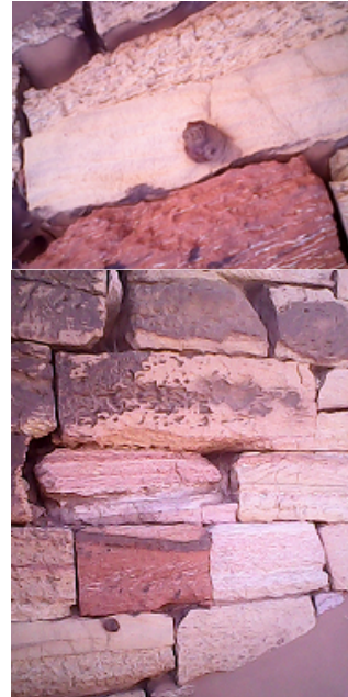
Figure 5b: The porous characteristic of sandstone. (Photo is author's own, 2015)
