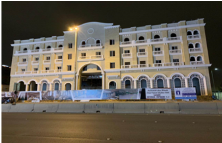
GFRG panels construction in Saudi Arabia
