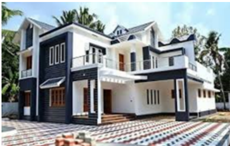
GFRG panels construction in Madurai
