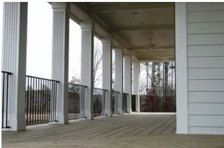
GFRG panels construction in Australia
