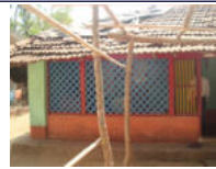
Figure 19: Wooden jali at building façade elevation
