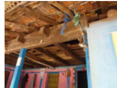
Figure 22: Vernacular roofing with thatch and Mangalore tile
