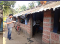
Figure 21: Laterite stone as building façade elevation material
