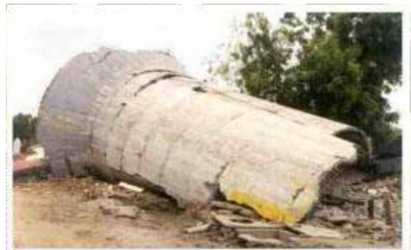
Figure 2: Collapsed 265 kL water tank in Chobari village, about 20 km from the epicenter of bhuj earthquake. The tank was approximately half full during the earthquake.
