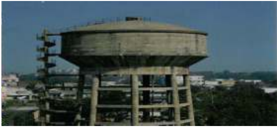
Figure 3: Intze Tank-Supporting on Columns
