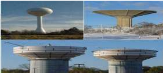
Figure 4: Intze Tank-Supporting on Shafts
