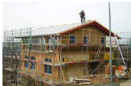
Fig-12 Straw bale wall can withstand great loads. Wall up to 3 stories can be constructed
