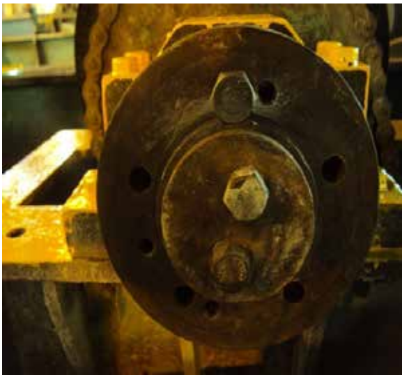
Figure7: Assembly unit shaft hub after make new tapping holes
