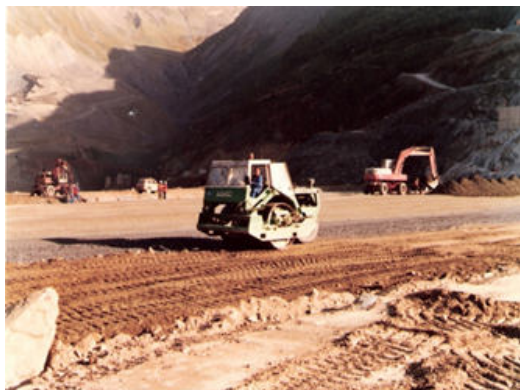
Figure 2: Poclair at the Grand'Maison dam first part, 140 m high, 10 m wide at the crest but 520 m at the base, 12.4 million m3 of fill had to be implemented (source ec1000.net)
