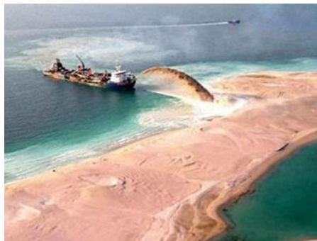
Figure 3: Construction of the Palm Island, the stage of Polderization; building a massive island, in the shape of a palm tree, until 2006. The island was to have a diameter of 5.5 km, increasing the coastline by 56 km. (Source adoutcivil.org)
