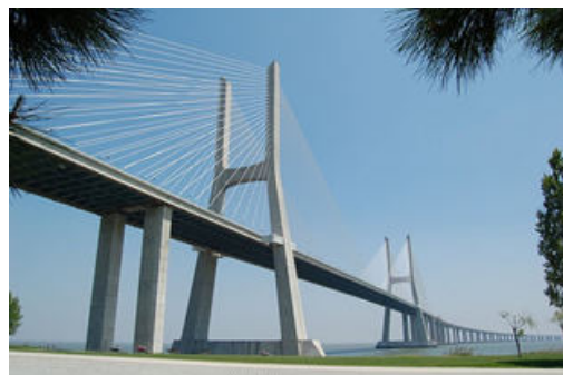
Figure 4: Vasco de Gama Bridge designed to withstand an earthquake up to 4.5 times stronger than the one that devastated Lisbon in 1755, which had then reached a magnitude of 8.7 on the Richter scale. It can also withstand winds blowing up to 250 km/h. (Source bonjourlisbonne.fr)
