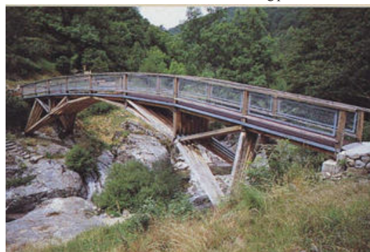
Figure 4: Picture of the Ajoux gateway in France
