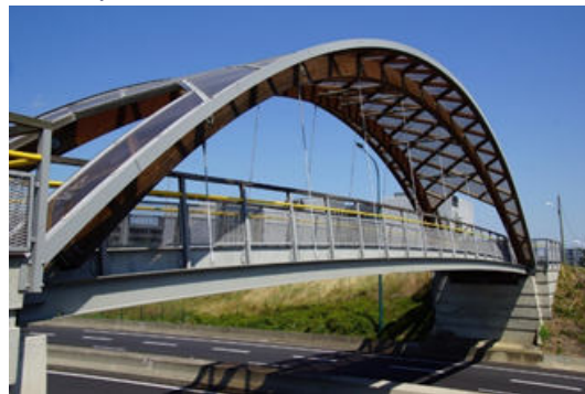
Figure 3: Picture of the Pinot footbridge in Blagnac
