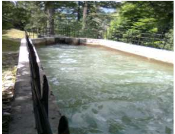
Figure 3: Desilting Chamber
