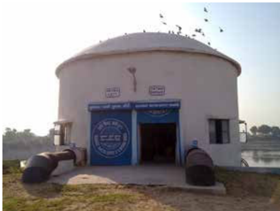
Figure-2 Pump House at Siddhi Sarovar
