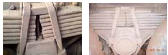
Fig.1- Whole stake failed from centre
