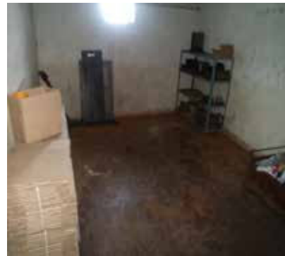
Photo5. Basement after sorting of material
