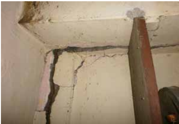
Fig. 2: Crack in column and beam junction
