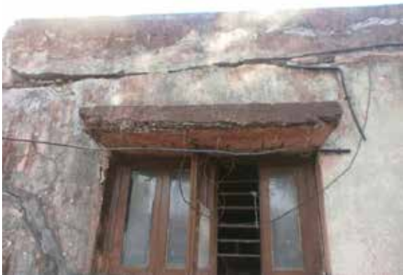
Fig.1 Cracks and exposed reinforced bar
