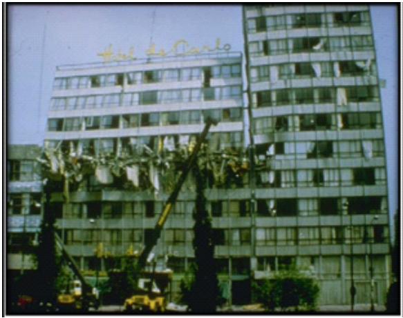
Figure 2: - Building collapsed due to Pounding
