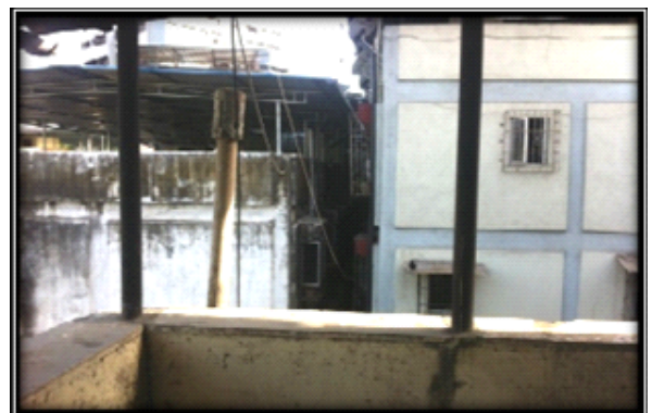
Figure 1:- Buildings close to each other (less than 10 ft. apart)
