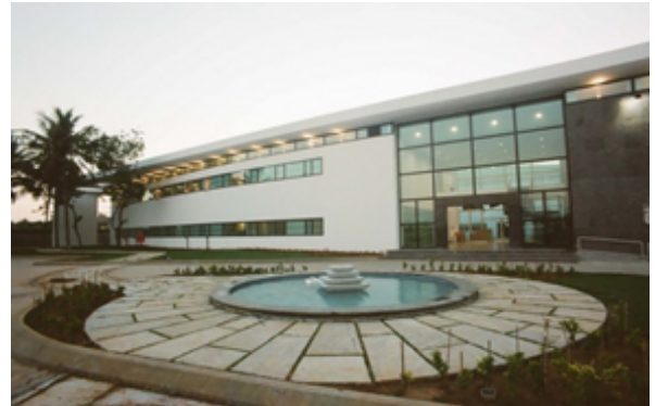
Figure 2. Thermal Storage at Grundfos Pumps, Chennai
