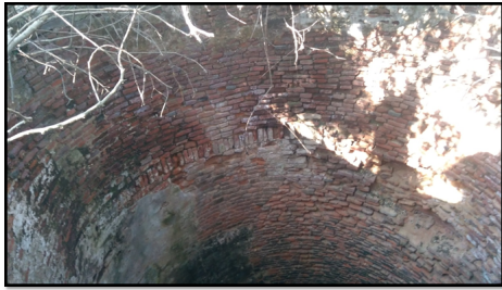
Fig 5 : Use of Lakhori Bricks in Well. [Photo Courtesy: Priyank Bharati]
