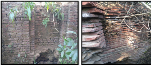
Fig 7 : Wall which shows rectangular niche. This type of niche was not used by Mughals. Mughals used arched niches not complete rectangular or square. Wall made of Lakhori Bricks (right hand side).[Photo Courtesy: Priyank Bharati]
