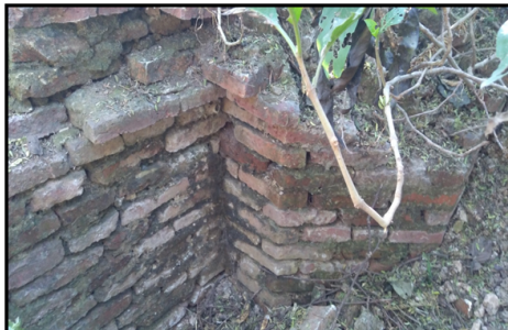
Fig 8 : Pillar like structure on the joint of some walls [Photo Courtesy: Priyank Bharati]
