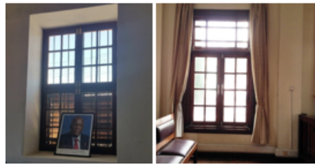
Figure 6 and 7; A window in the Old Boma and Court of Appeals buildings.
