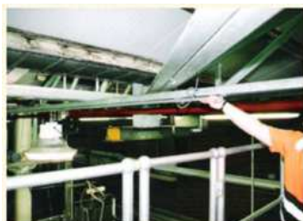
Sliding lighting systems. Photo: J.Culvenor, thanks to Fosters/CUBI
