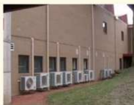
Air-conditioning systems located at ground level with good access. Photo: J.Culvenor
